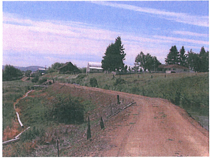
Westside Ditch – Please Note Elevation
